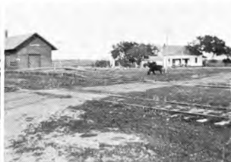
Northwestern depot at Sawyer and the Manning residence (1926)
