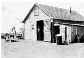
R. W. Wirz repair shop at Sawyer (1926)
