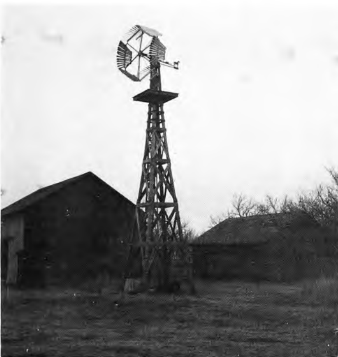
Photo from Guy Brown, Jr. Early-day windmill with wooden tower and wheel. This was a "self-closing" type, especially suited for the high winds of the prairies. Instead of a flat wheel facing into the wind, the wheel was made of several sections forming a shallow cone facing away from the wind. As wind speeds increased, the "wings" folded forward to take less wind and so keep the windmill from racking itself to pieces or overpumping. The wings could be completely closed by a lever from the bottom; this one is shown in the closed position.
