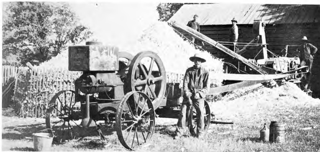
Shelling corn, about 1917, with a Sandwich 4-hole sheller and a 10-HP Water Lou Boy gasoline engine. The man sitting on the engine wheel is Charley Nichols.
