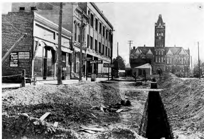
Photo from Geneva State Bank Laying steam pipes to heat courthouse and business houses (about 1910).
