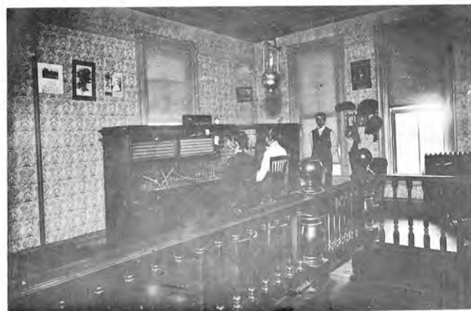
Photo from Geneva State Bank Early telephone switchboard. Left to right: Laura Bender, operator; Kate Porter; Monroe Heisey, trouble man.
