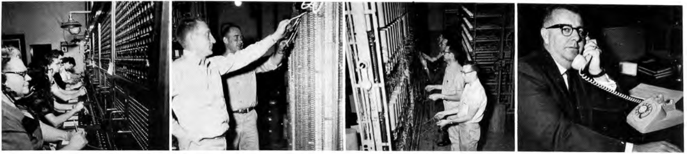
The shift to the dial system (1963). Left: Switchboard before pulling picks for dial system (Miss Emma Ebbeka in foreground). Second picture: Pulling picks in old office—L. D. Anderson ( left ) and Roger Bates. Third picture: Pulling picks to make change from operator switchboard to dial system. The second man from the front is Lowell Garrett of the Geneva exchange; the other three are from the Lincoln office. Fourth picture: Mayor Francis McPeck making first dial call to Commercial Supervisor in Lincoln.
